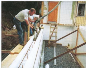
Raskas betonivalu kevyesti pumpulla
